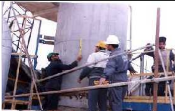
Checking fitting of new section
