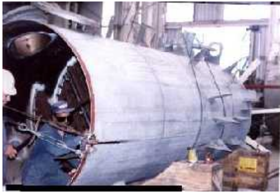
Adjusting diameter of new section
