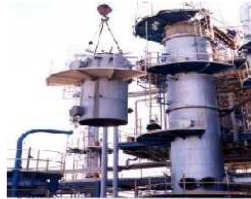
Replacing top section
