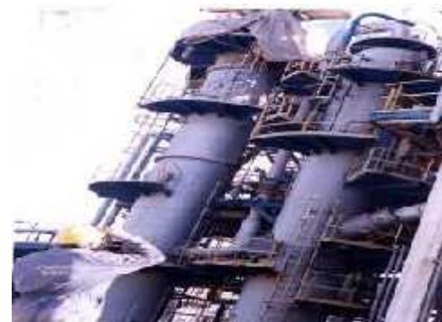
After assembling top section
